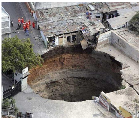
Sinkhole in Guatemala City
